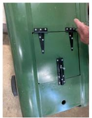
Cut the bottom edge of the door and install the sliding bolt using the M5 bolts.
